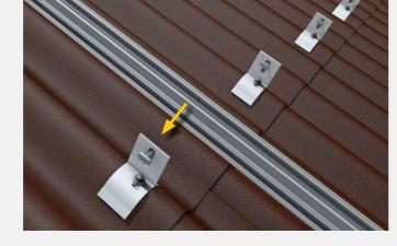
2. Mounting the vertical universal profile (UP-X) The pre-assembled universal profiles are then securely screwed onto the TS-COR using the M10 hammerhead screw.
