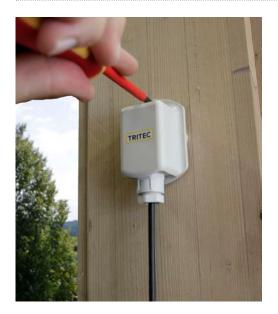
To ensure maximum accuracy of the measuring result, the outside temperature sensor must be fitted at least 2.5m off the ground on a flat surface. Installation close to windows, doors or steam outlets may falsify the measuring result.
